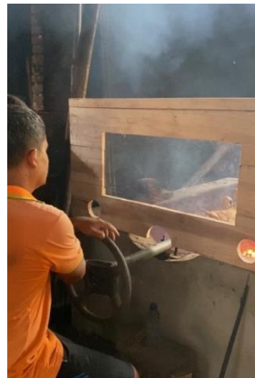
Figure 1. The Rolling Process After Repair With the Installation of Cross-Wood Boards
