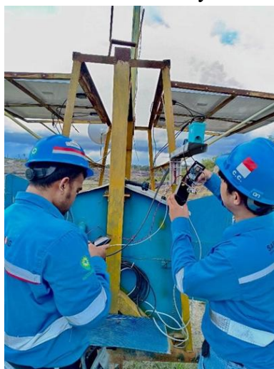
Figure 9. Rainfall and Water Level Sensor Assembly
