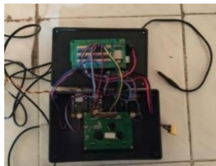
Figure 6 Installing a TDS Sensor Device with Arduino Mega
